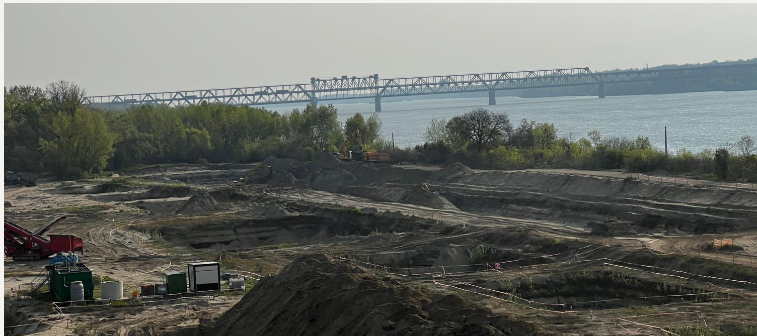
Earthworks and site preparation for the production complex
