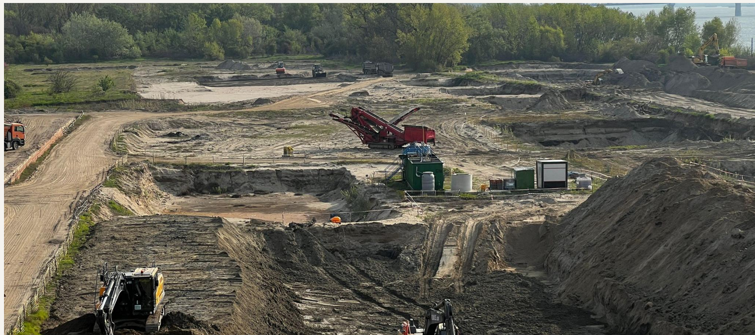
Heavy excavation preparing foundations for industrial structures
