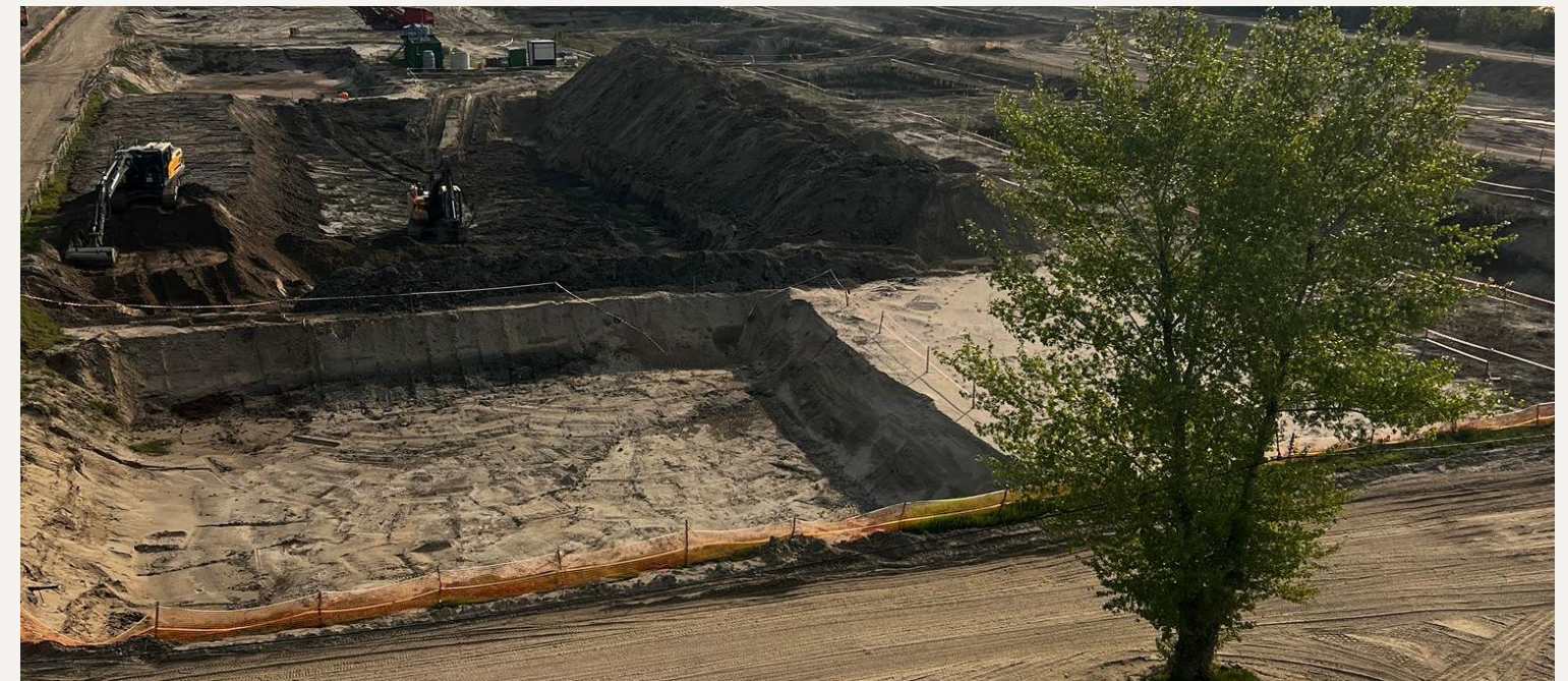
Construction equipment mobilized on site
